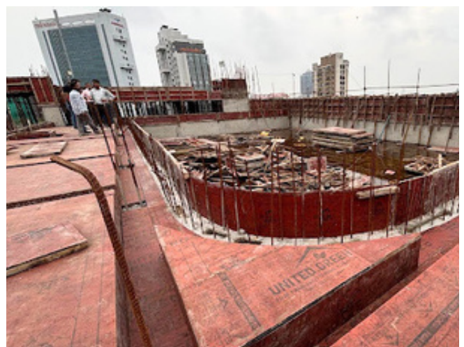
4th Floor Above Roof Work Images
