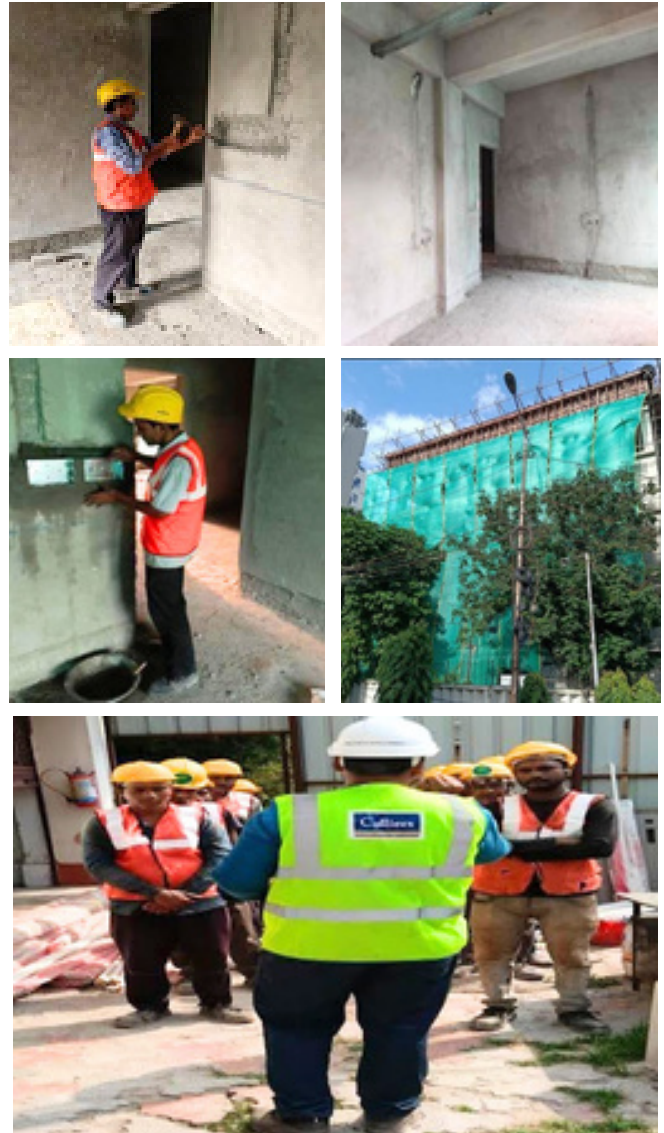
MEP Work Images - Work In Progress
